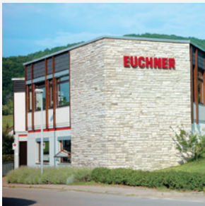
Production location in Unterböhringen
