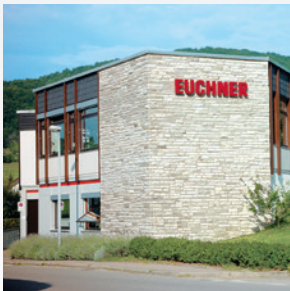
Production location in Unterböhringen
