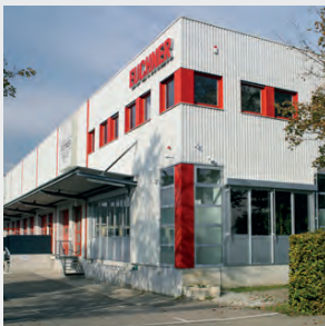
Logistics center in Leinfelden-Echterdingen
